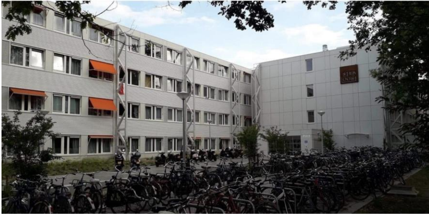
Figure VII: A former hospital now used as housing at Stek Oost, Amsterdam Oost
