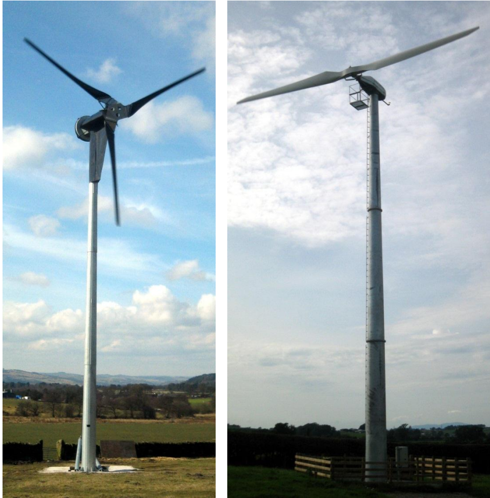
Figure 3 The two small wind turbines monitored and modelled in this paper; the Proven 35-1 (left) and Gaia-Wind 133 tubular tower (right).
