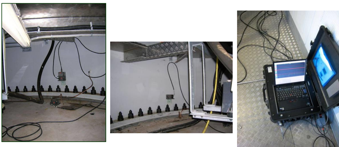
Figure 5. Installation of Guralp CMG-5U uniaxial accelerometers in Turbine 1.
