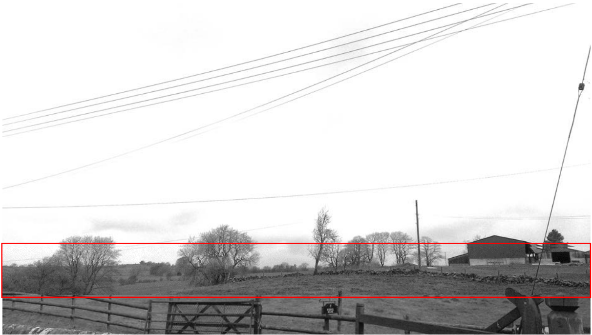
Figure 1. Damaged dry-stone walls
