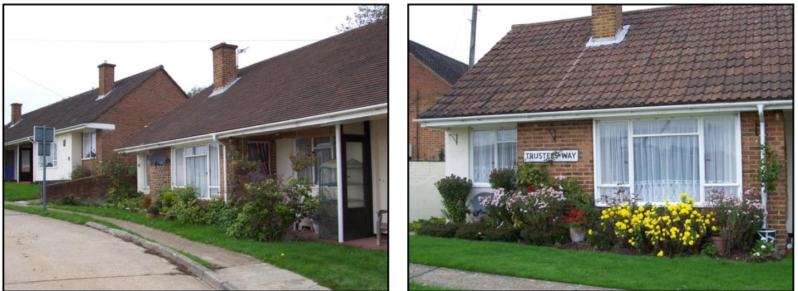
Figure 5.4 and Figure 5.5: Bungalows in the old village
