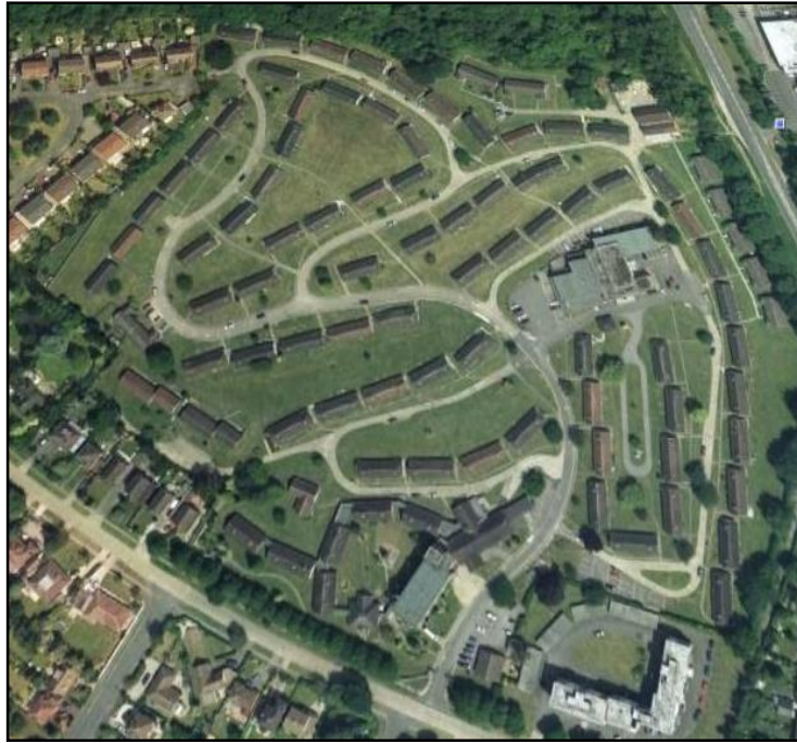
Figure 5.9: Aerial view of the old village
