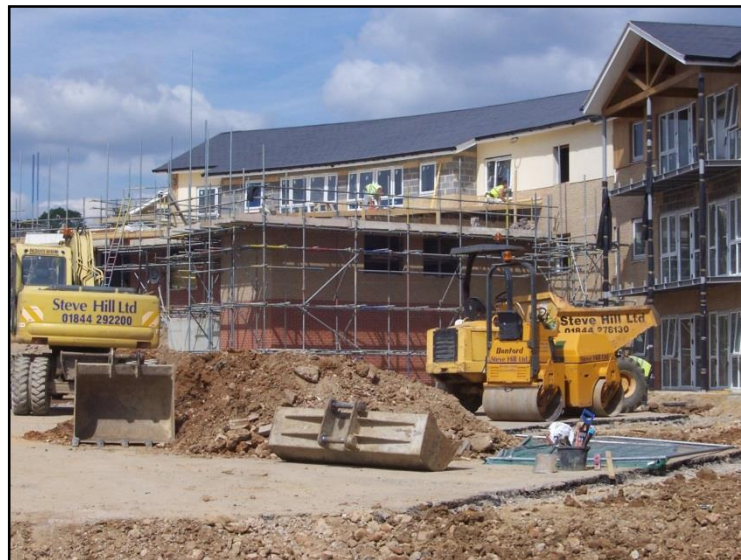
Figure 5.15: Construction of new apartments
