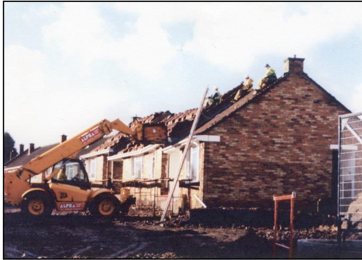
Figure 5.14: Demolition of old village buildings
