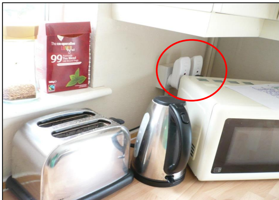
Figure 4.5. Two EDF Transmitter Plugs (IAMs) installed in kitchen
