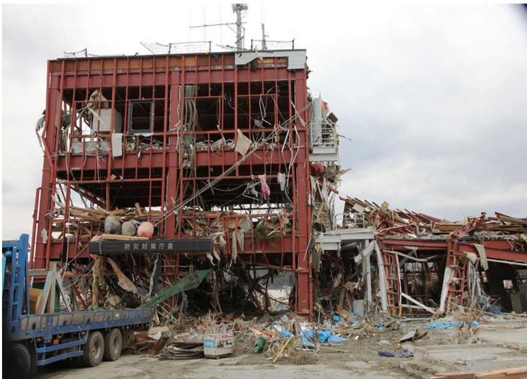
Figure 28: The former Disaster Prevention Centre
