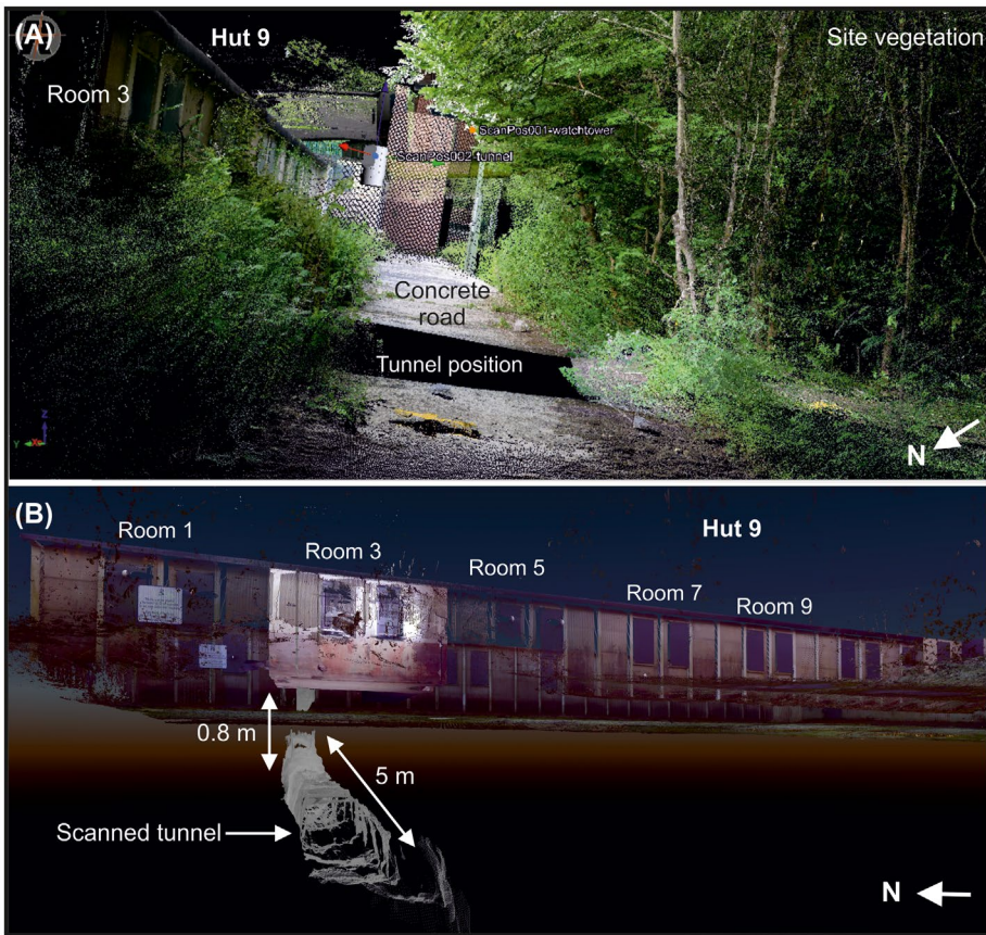
Figure 11. Digital screen-grabs of ground-based LiDAR data-sets acquired onsite. (A) Surface data-set showing approximate tunnel position and (B) Tunnel data-set with merged Hut, room and tunnel scans shown. See supplementary data for digital fly-throughs.
