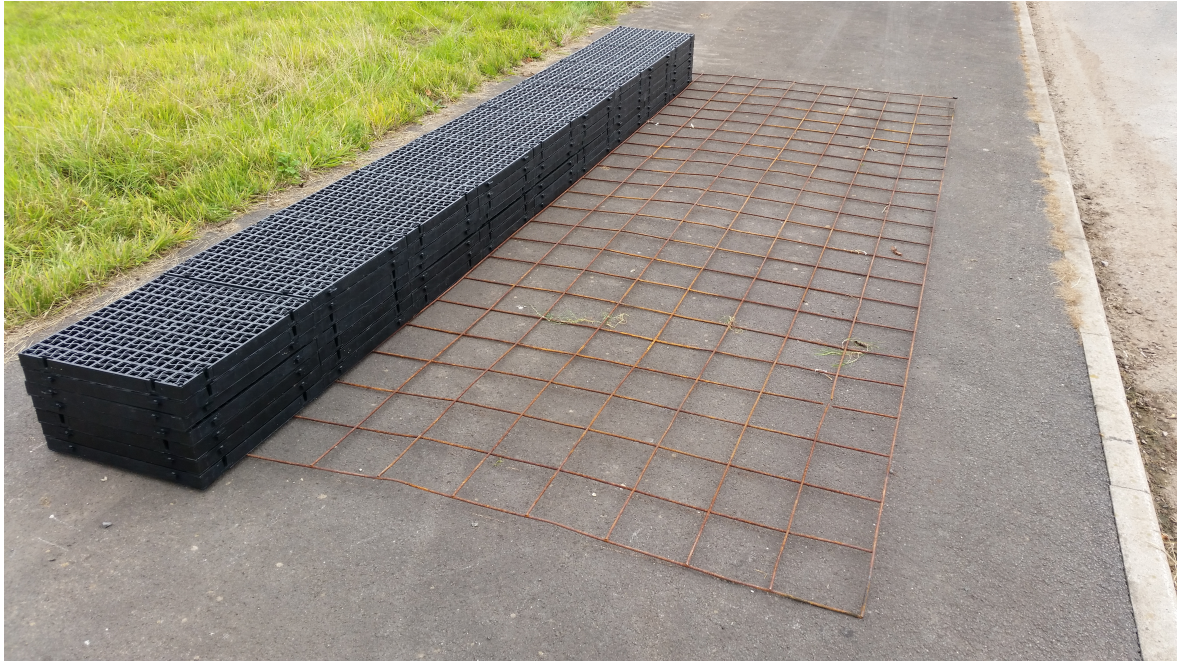
Figure 3.11: The data fusion testing mesh, with the plastic grids in position and giving a simulated cover depth of 280 mm.
