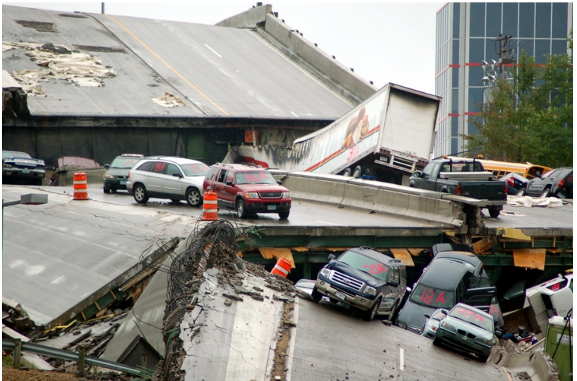
Figure 1.1: The aftermath of the I-35W bridge collapse in 2007 (from Rofidal [17]).
