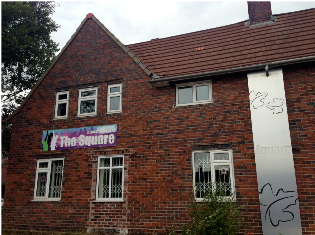
Figure 2: Meir North's community centre
