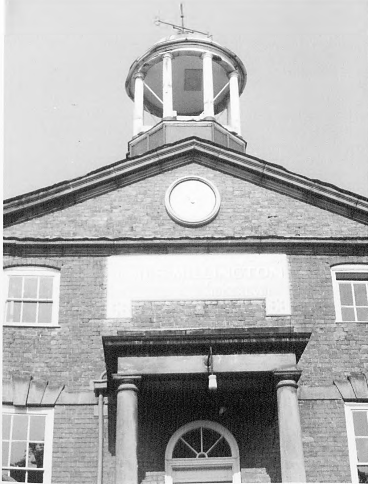
Plate 15: Millington's Hospital School, Shrewsbury (est.1748)
