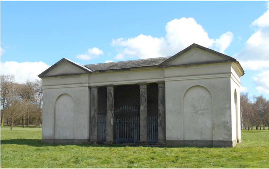
Figure 2. The Sulphur Bathhouse, Kedleston. Image: Author
