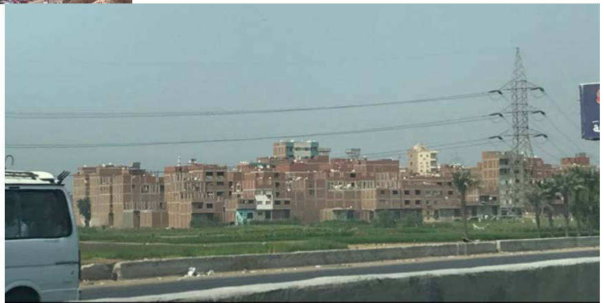
Unplanned growth on agricultural land (Source: author's site visits [5]).
