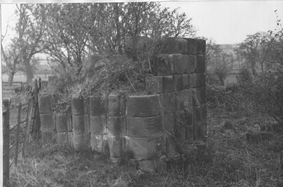
(a) One of the piers of the central crossing.
