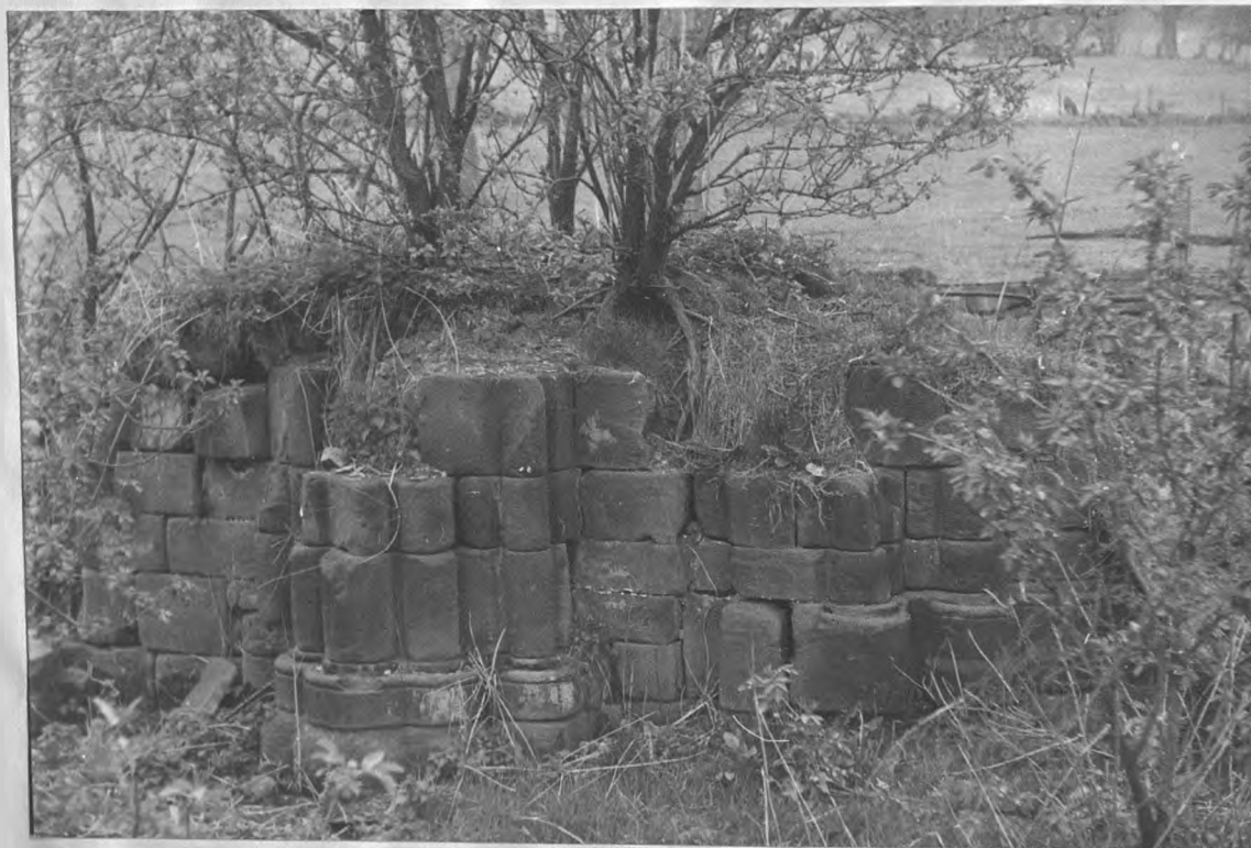
(b) Part of the north wall of the Nave.
