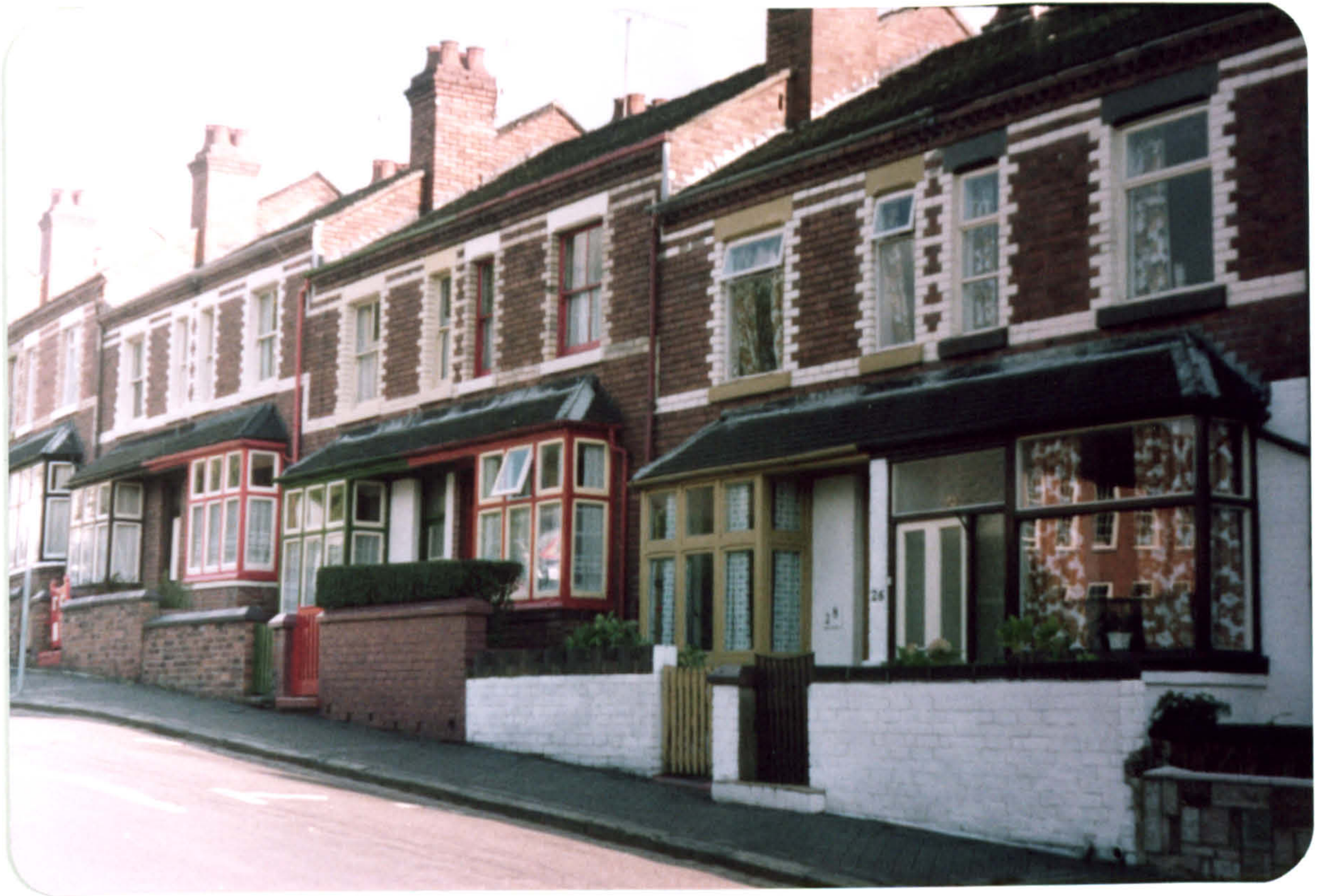
Figure 4.51 A view of sub-divided Victorian housing at Newcastle
