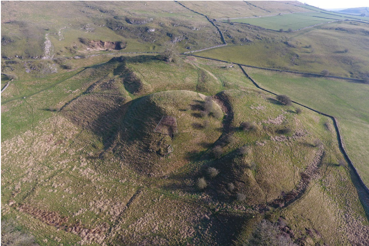
Figure 3.13: Oblique aerial view showing the hollow-ways, possible field or canal boundaries, and the wider earthworks at Pilsbury Castle, February 2020 (Image credit: Dr Alex Nobajas/Helen Malbon).
